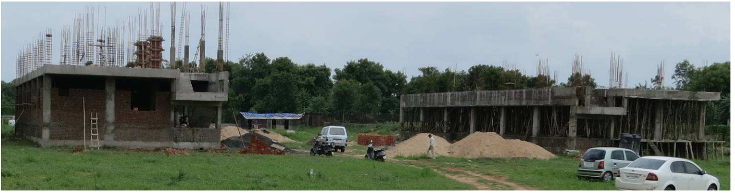
GUJARAT, The two buildings are taking shape on our own two acres.
