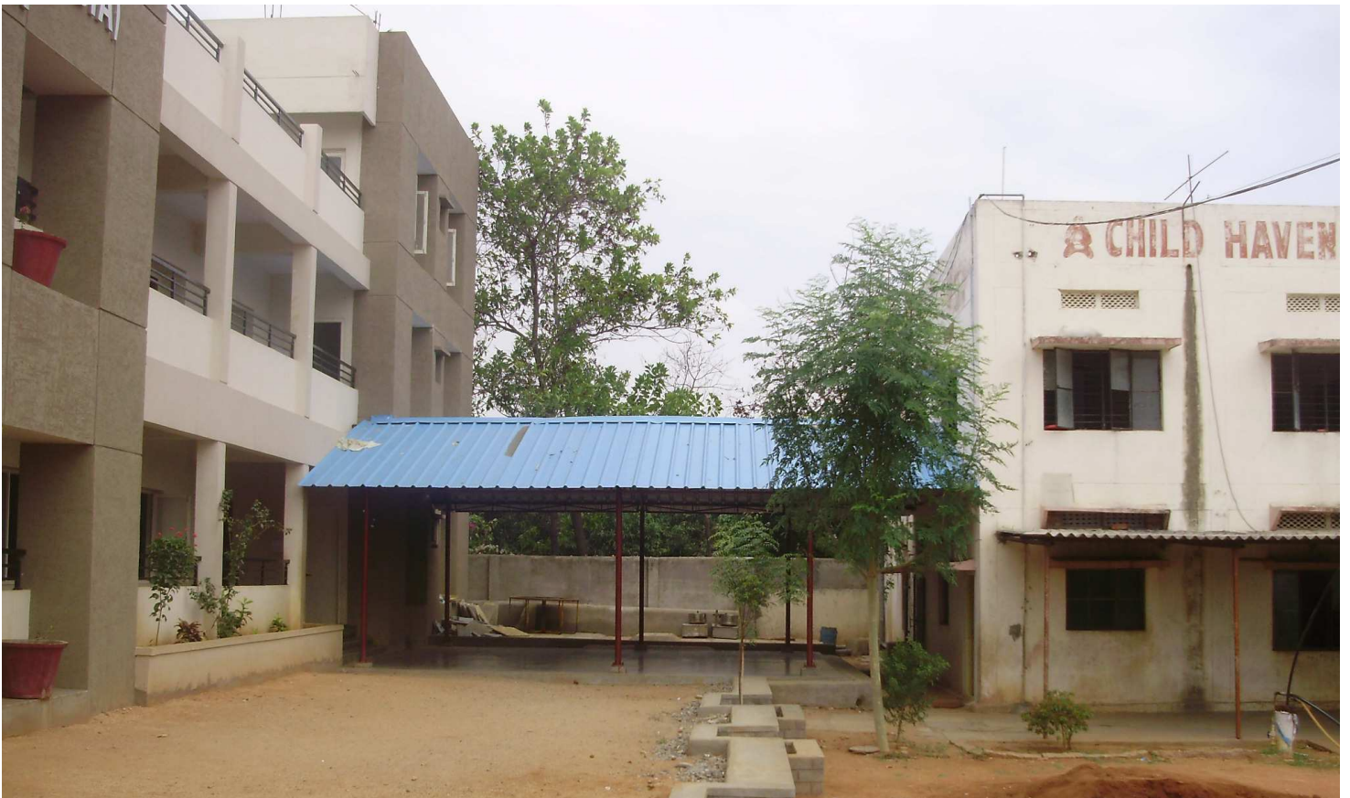
HYDERABAD, The Oceanside Child Haven Support Group in Qualicum Beach, B.C. put up the initial money to construct this much-needed passage way (about 20x25 feet) between the new building, left, and the old building. It also serves as a shady study hall.
