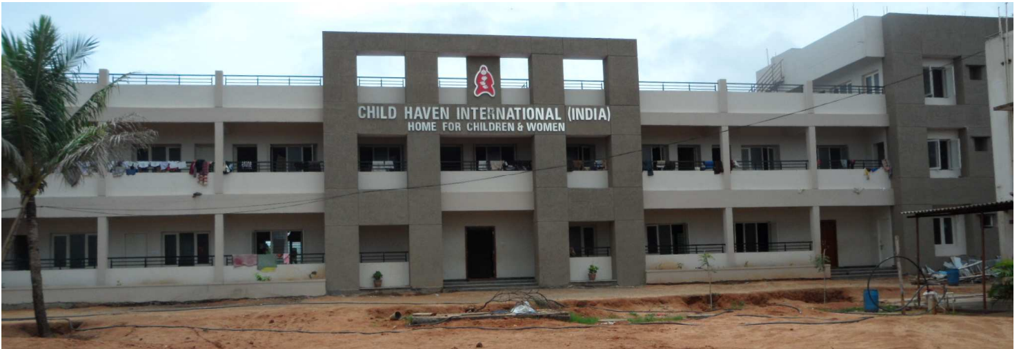
HYDERABAD – Completed new building, with boys Dorm, office space, Assembly/Dining Hall.
